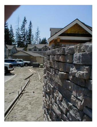
The picture to the left is a violation and shows an example of a stone wall that enhances climbing. Bricks, support posts, and similar construction must not provide hand or foot hold for climbing.
