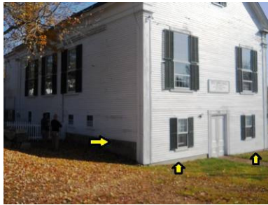
Uninsulated Foundation / Slab
