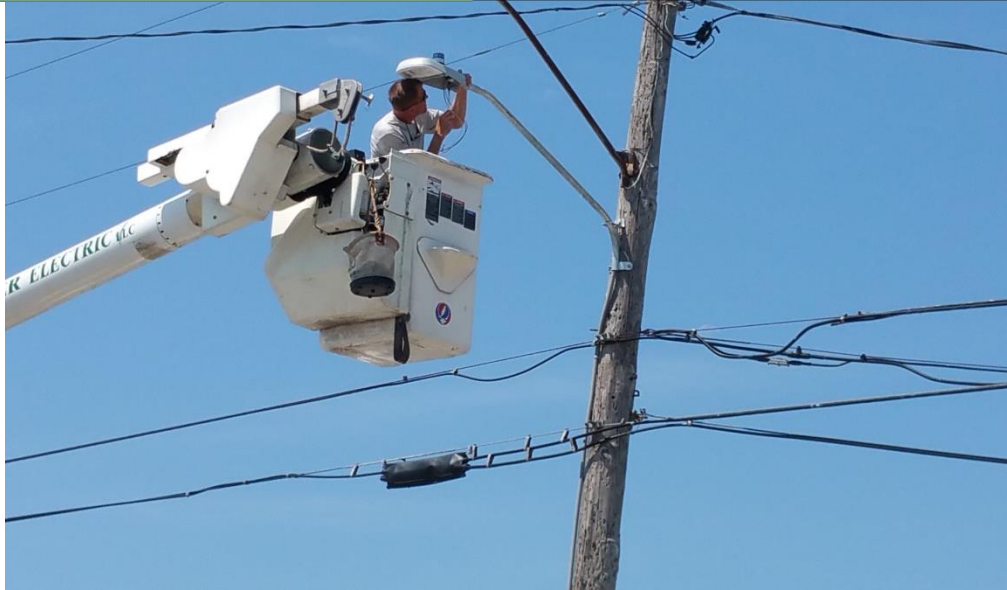
Figure 1: Test LED Streetlight being installed at the corner of Perkins Rd. and Ocean Blvd. in June
