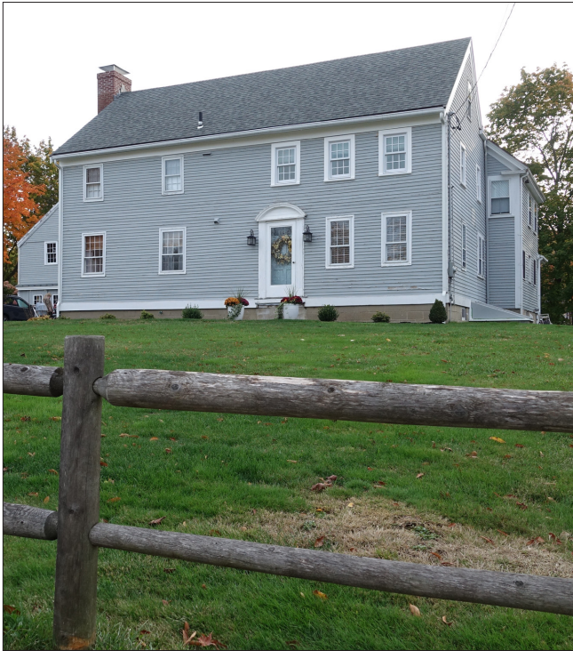
This 2 1/2-story Colonial residence has a 2-story addition to the right and a one-story addition to the left. The form, scale, materials, and detailing are similar, but subservient to the main block allowing the historic portion of the house to maintain its prominence from the streetscape.
