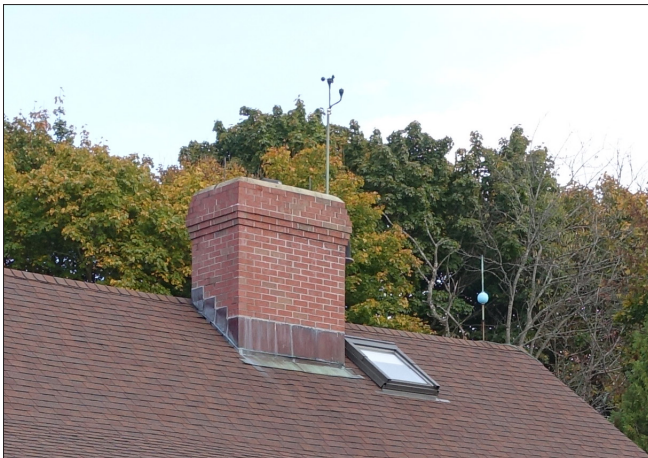
The skylight has a low profile and parallel to the roof slope, minimizing its visibility. Also note the stepped copper flashing at the brick chimney.
