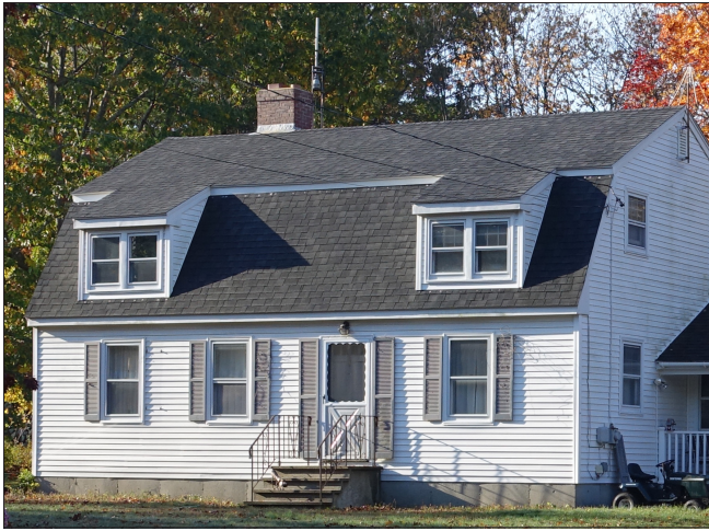
Gambrel roof forms are relatively rare in Rye. However, chimneys are often located at or near the roof ridge.
