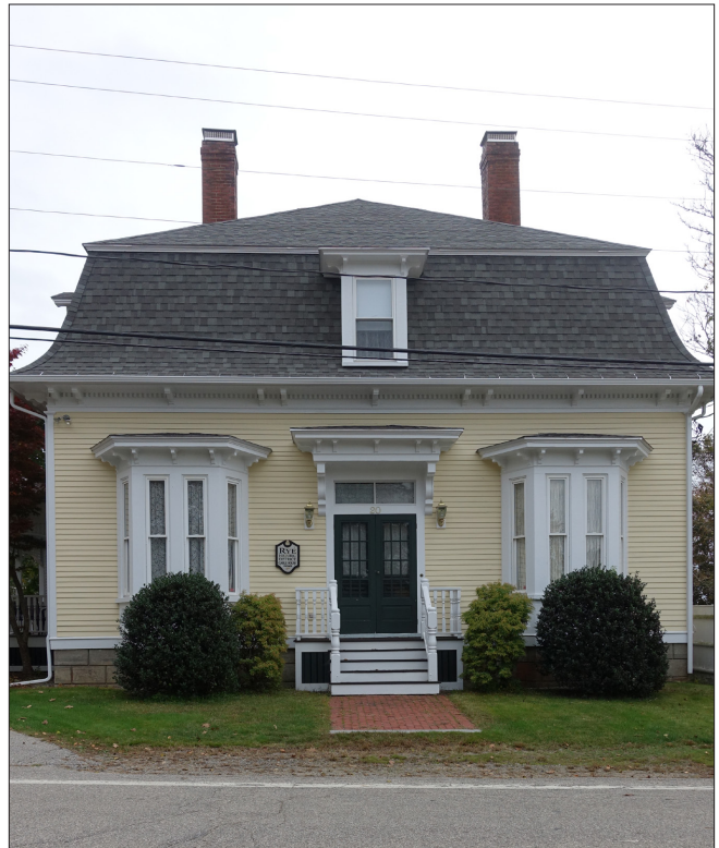
Roof forms can provide a dramatic building silhouette against the sky. In this case, the Mansard roof, typical of Second Empire buildings, has deep projecting eaves and two, symmetrically placed chimneys, as on the historic “Cable House” above.
