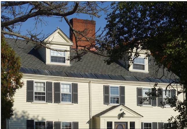
Gable roof dormers can typically be found at early Federal and Greek Revival, and Colonial Revival buildings. This example is pedimented and includes 8/8 windows. Cheek walls on dormers typically have wood clapboard cladding. Also note the massive, central brick chimney and metal ice shield along the eave.
