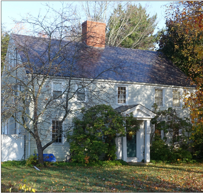
Slate roofing is often found on Rye's older buildings. Also note the massive central chimney.
