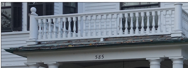
Copper is a traditional metal roofing material that does not require painting. The standing seams, as shown in this example, create a regular pattern along the roof surface.
