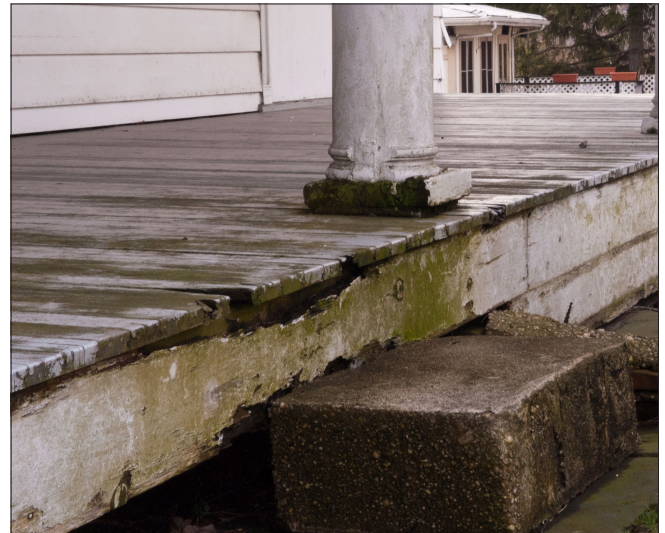
Porches, steps and other areas where the woodwork is laid horizontally or located close to the ground are often the first to deteriorate. Ongoing exposure to moisture can lead to rot of the column bases, porch deck and apron.
