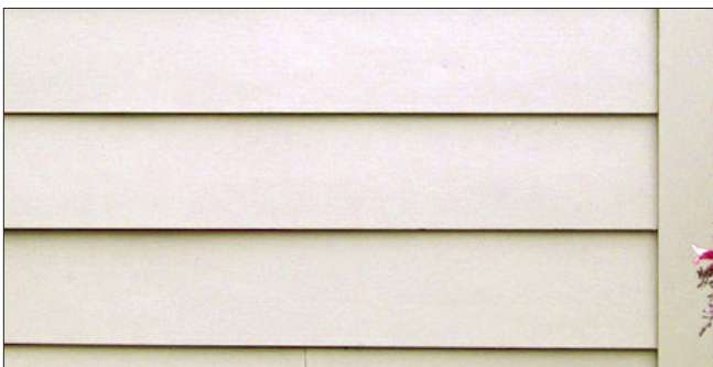
Fiber-cement siding and trim generally do not have the same dimensions as traditional wood elements including the width of corner boards and the depth of individual clapboards. This results in visual differences when compared to wood siding.
