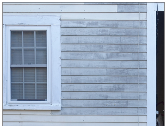
Selective replacement of deteriorated woodwork should endeavor to match the visual characteristics of the historic woodwork in dimension, profile, and materials.
