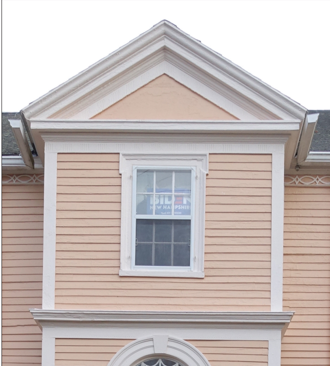
Clapboard siding can be found at the wall surface while flush siding is located in the pediment. The narrow spacing of the siding enhances the shadow lines on the wall surface.
