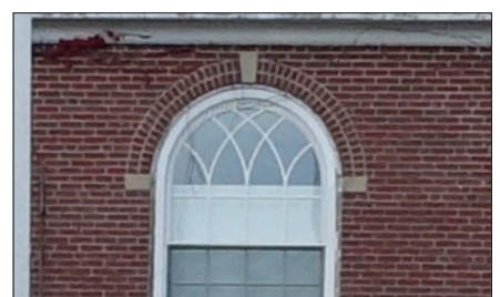
Limestone - A sedimentary rock; used for building walls, window sills and lintels, ornamental stone trim and sculpture.
