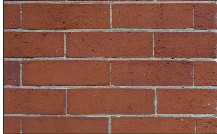
20th Century Brick - A hard, dense, fired-clay, regularly shaped building component; sometimes with a glazed surface.
