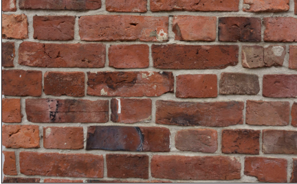
18th-19th Century Brick - A soft, fired-clay, fairly regularly shaped building component; often with color and surface variations
