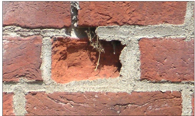
The surface of the center brick has spalled. The repointing mortar is harder than the brick and likely includes too much Portland cement. The mortar should be completely replaced with softer mortar.
