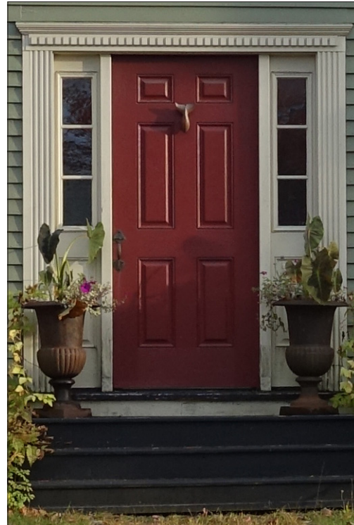
This wood paneled door has simple three-light sidelights.
