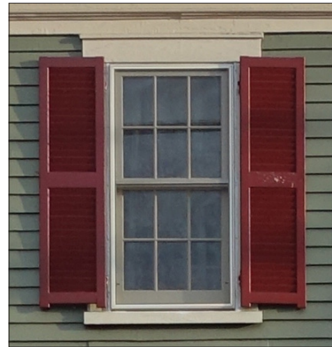
The majority of historic windows in Rye are double-hung, made of wood, and are in a 6/6 configuration. This example also includes wood louvered shutters that are operable and sized to fit the window opening when closed.
