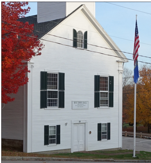
Town Hall includes a variety of wood windows including a 6/6 arched head window at the gable end and monumental 20/20 double-hung windows at the second floor, all with operable shutters.
