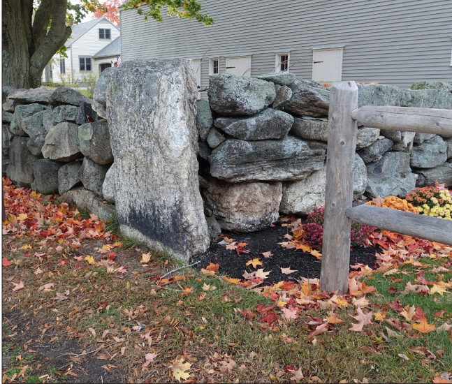
Granite, which is readily available in Rye, is a very durable material that is ideal for the construction of landscape walls. This dry-laid granite wall includes larger stones held in place by smaller ones, all topped by a relatively flat capstone.
