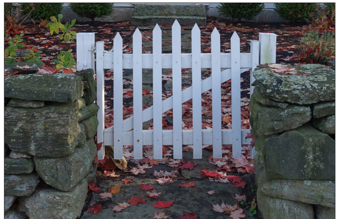
Gates at wood fences tend to reflect the pattern of the fencing. Paired gates are typically used at larger openings.
