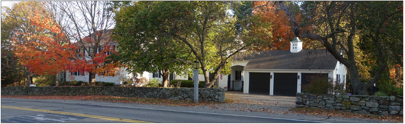
Additions should include forms, proportions, trim, details, and materials similar to the historic portion of the building.
