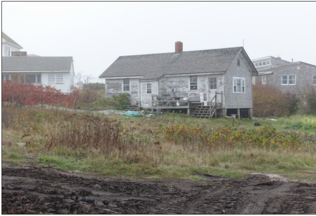
Zone 4 includes support buildings are largely simple framed cottages.
