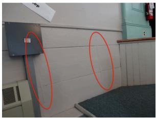
Figure 48: Detail of 1839 dadoes in the original sanctuary space of Rye Town Hall, showing filled-in pew mortises.
