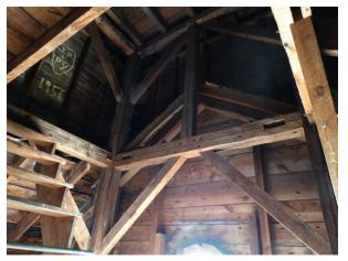
Figure 40: View of bell-tower drum framing looking up and south, showing 1873 framing with salvaged 1839 timber elements.
