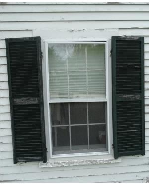
Figure 74: Detail of typical modern replacement shutters, which exhibit warping and minor deterioration.
