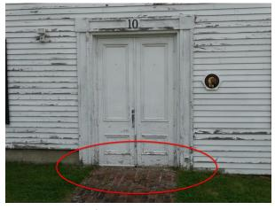
Figure 72: Detail of original west, main entrance showing area of grade to be lowered and trim and original doors to be consolidated with epoxy.
