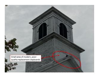
Figure 76: View of tower looking southeast, showing predominantly original clapboards and trims, with some later, low-quality replacements (indicated in red).
