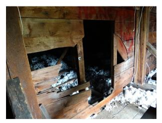
Figure 39: View of attic: 1839 gable facade, encapsulated in the 1873 front expansion, showing opening for the original demi-lune fan gable detail, and footprint of the original eaves fascia.
