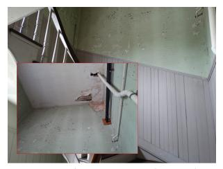
Figure 85: View of north staircase wall (Room 202) looking north, showing deteriorating paint and original plaster. Inset: View of ceiling above (Room 302) showing failing plaster, to be conserved and repaired.
