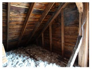
Figure 87: Detail of attic space above Room 302 showing 1874 balloon framing and recent cellulose insulation.
