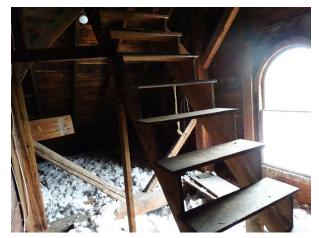
Figure 88: Detail of attic space above Room 302 showing original 1870s staircase accessing the bell tower.
