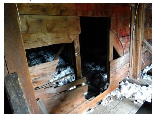
Figure 55: View of the 1839 front gable, encapsulated within the west addition of 1873. Note the sheathing divested of clapboards, and the rough opening for the original demi-lune gable feature.
