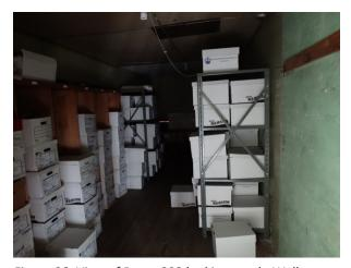
Figure 86: View of Room 302 looking south. Wall plaster is intact and requires stabilization. Most of the ceiling plaster has been reinforced with modern drywall.
