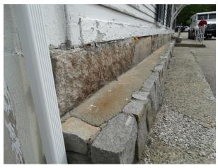
Figure 70: Detail of the composite stone, brick and concrete foundation, south elevation looking east, showing re-pointing in 2011.
