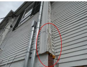
Figure 77: Detail of corner pilaster base, east end of main building south elevation, showing poor past repairs and spray-foam insulation.
