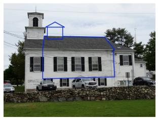
Figure 46: Annotated view of Rye Town Hall looking north, showing the proportions of the 1839 church within the current structure.
