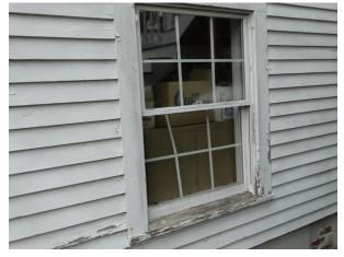
Figure 81: Detail of modern window, east elevation, ground floor, showing broken false muntins.
