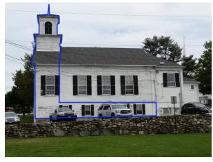
Figure 52: Annotated image of the Rye Town Hall looking north, showing the lines of the ground-floor, front and tower additions made in 1873.
