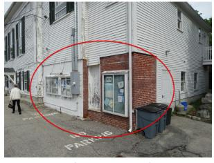
Figure 79: Detail of southeast corner of south and east elevations looking northwest, showing brick vault and privy foundation.
