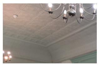
Figure 64: View of embossed metal ceiling covering installed in 1912 to cover the original 1839 plaster tray ceiling.
