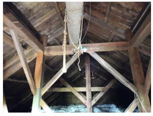
Figure 50: View of 1839 bell tower queen-post trusses, attic looking east and cut off at the top in 1873 when the original tower was removed.
