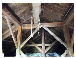
Figure 37: View of main attic looking east, showing cutoff trusses that supported the 1839 bell tower before it was moved forward (west) in 1873.
