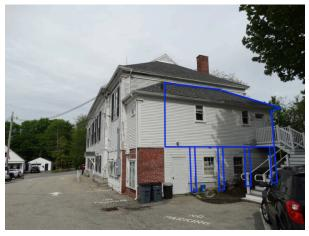
Figure 61: Annotated view of Rye Town Hall, east elevation looking northwest, showing the configuration of the 1911 second-floor porch addition and brick piers.
