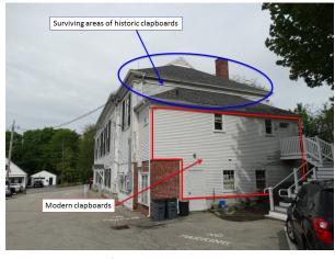
Figure 80: View of east elevation looking northwest, showing areas of original clapboards and trims (blue), and modern replacements (red).
