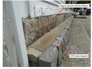
Figure 78: Detail of south elevation foundation looking east, showing original foundation and later retaining wall with recent mortar repointing.
