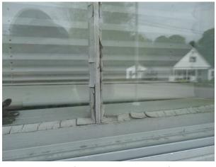
Figure 73: Detail of typical window glazing failure.
