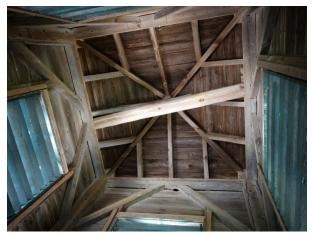
Figure 41: View of belfry looking up and to the east, showing framing scheme.
