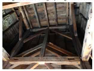
Figure 54: View of 1873 bell tower framing, looking west. Note the mix of out-of-context, reused 1839 timbers (random, abandoned mortise joints, and both hewn and sash-sawn elements) compared to the circular-sawn elements from 1873.
