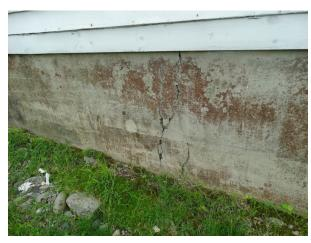
Figure 84: Detail of concrete foundation, north elevation, showing typical cracks, non-structural.
