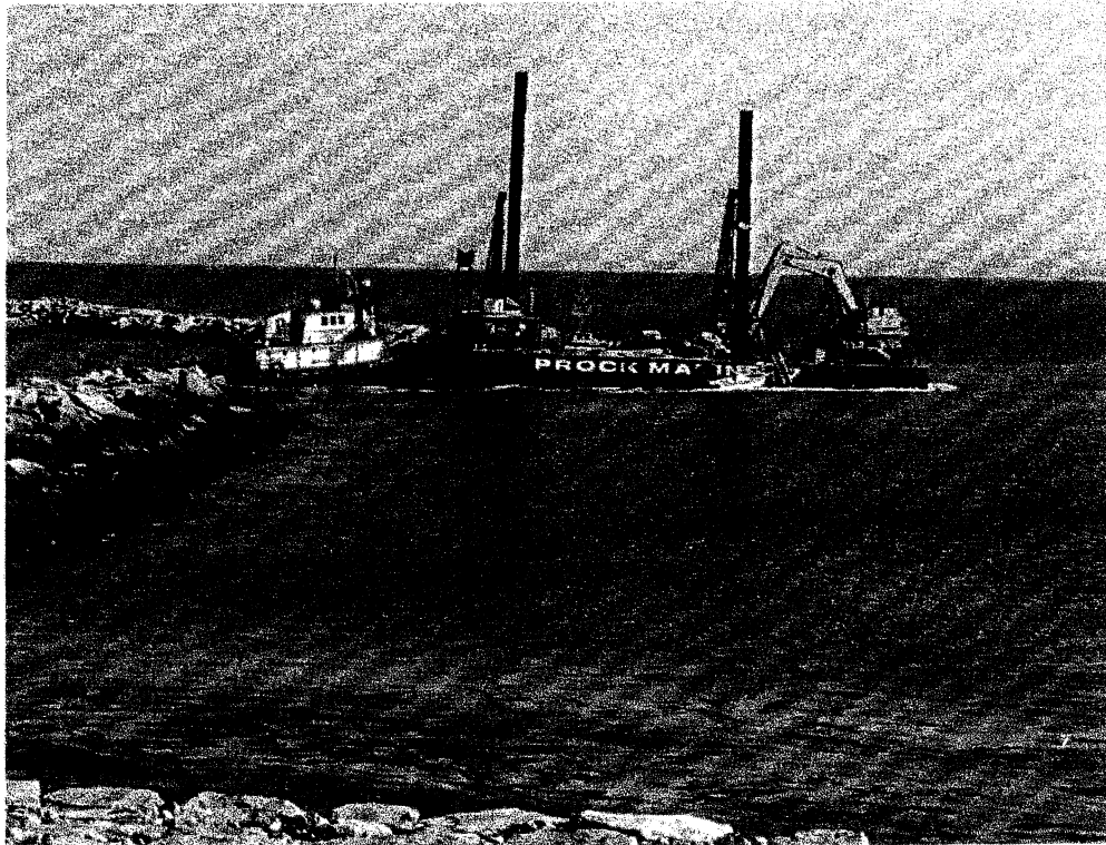
(The Prock Marine dredge equipment departing Rye Harbor after completing their four months of dredge work. Rye Harbor finally dredged after 30 years. Photo by Mae Winslow)
