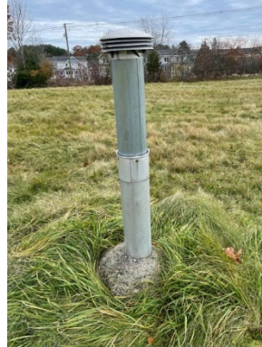
Photo #2 - Repaired gas vent in November 2021.
