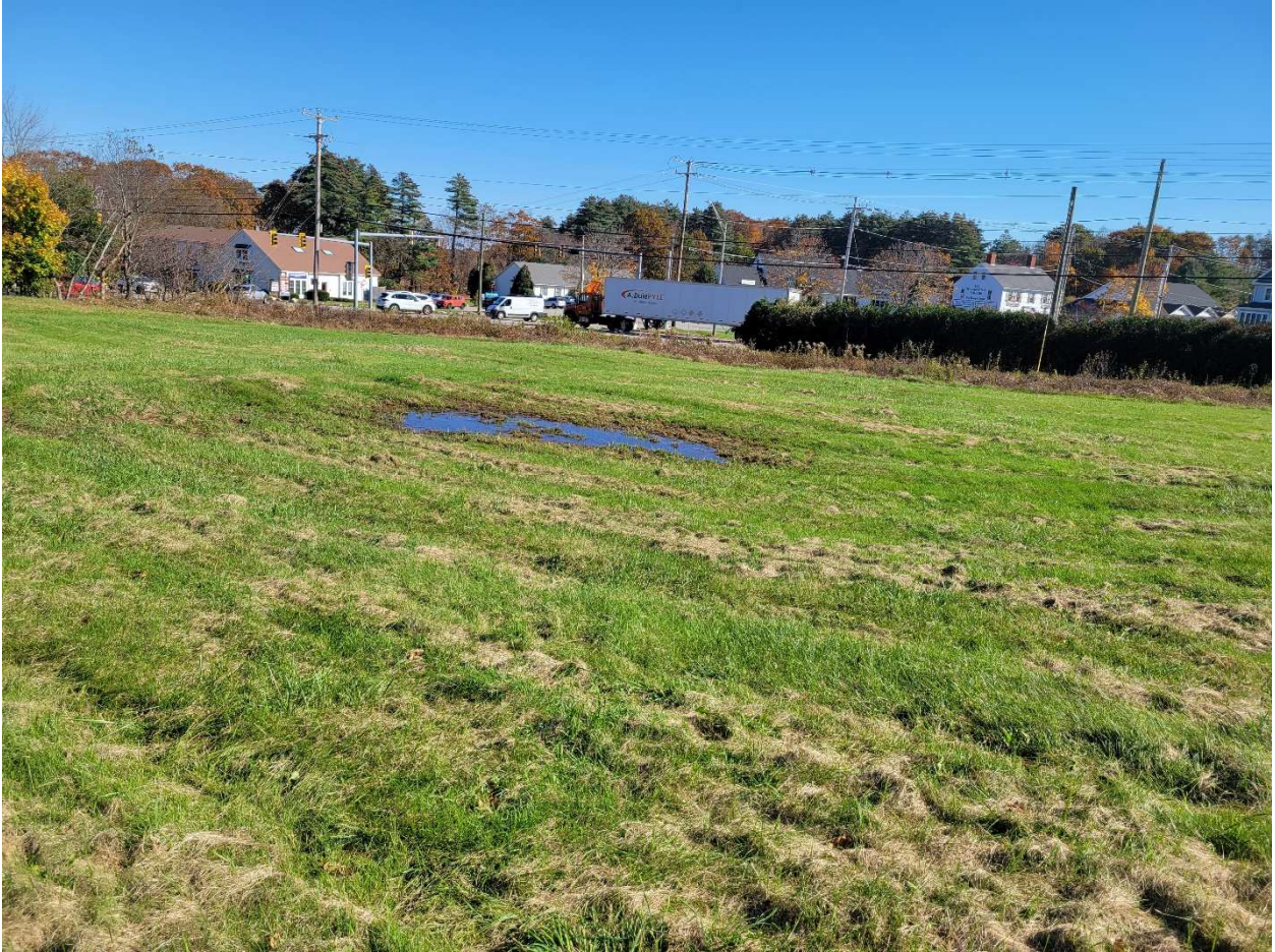
Photo 1: Low spot with standing water
