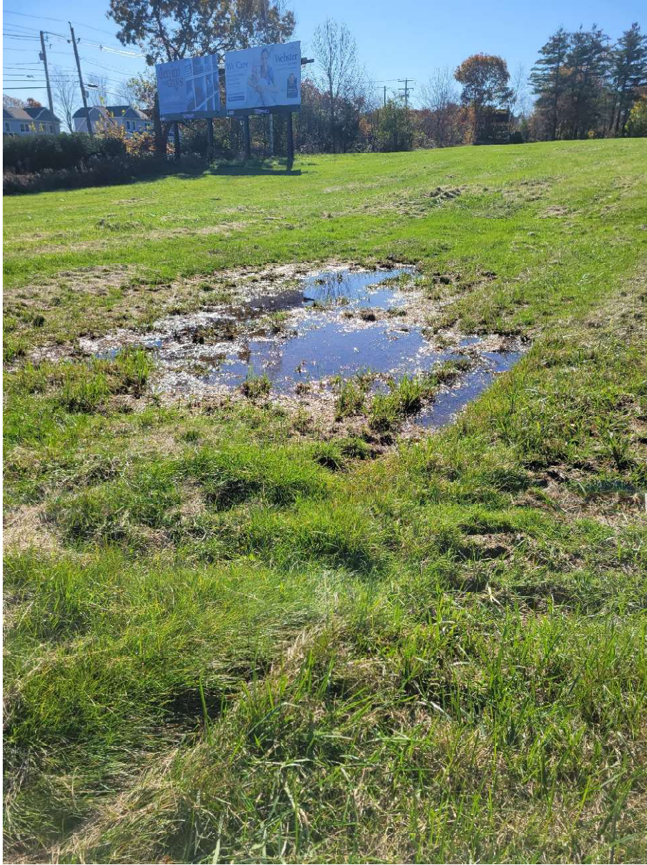
Photo 2: Low spot with standing water
