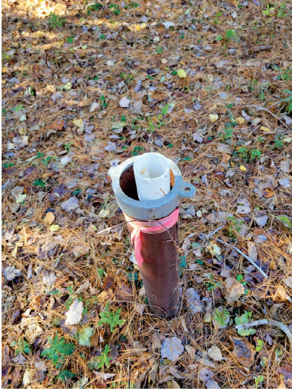
Photo 1: PVC riser sticking out of casing MW-101
