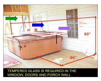
Tempered glazing is required in walls and fences enclosing indoor and outdoor swimming pools, hot tubs and spas where the bottom edge of the glazing is less than 60" above a walking surface and within 60" horizontally of the water's edge.
