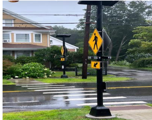
New LED Rectangular Rapid Flashing Beacons at
