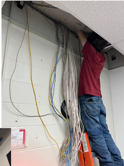
Old Wiring being pruned out
