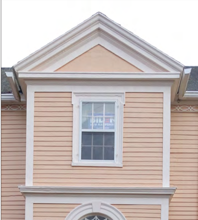
Clapboard siding can be found at the wall surface while flush siding is located in the pediment. The narrow spacing of the siding enhances the shadow lines on the wall surface.
