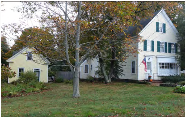
The HDC seeks to maintain the historic character of Rye's designated historic properties. Regular maintenance is encouraged at all buildings, outbuildings, and structures.
