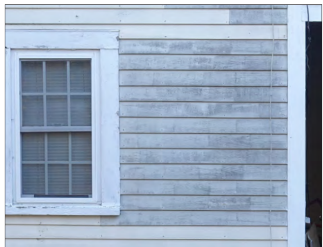
Selective replacement of deteriorated woodwork should endeavor to match the visual characteristics of the historic woodwork in dimension, profile, and materials.
