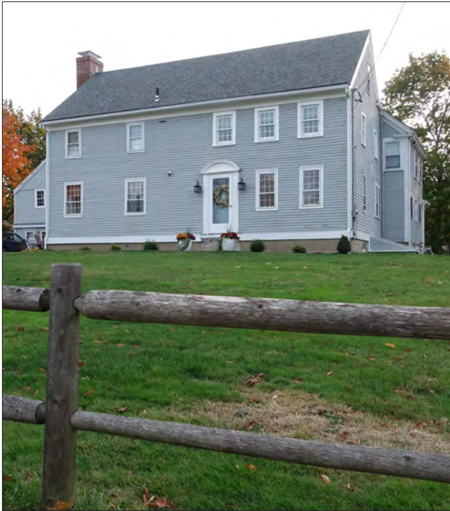
This 2 1/2-story Colonial residence has a 2-story addition to the right and a one-story addition to the left. The form, scale, materials, and detailing are similar, but subservient to the main block allowing the historic portion of the house to maintain its prominence from the streetscape.
