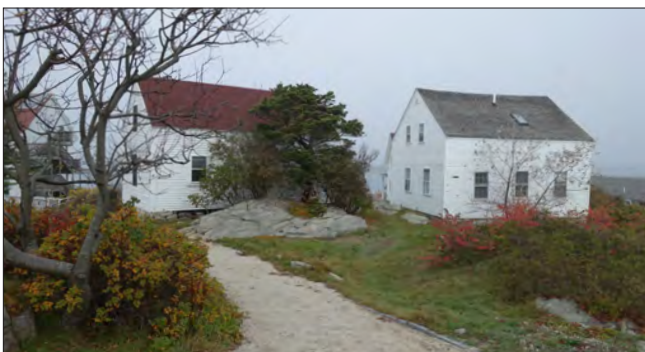
Zone 1 includes support buildings south of the Hotel Complex.
