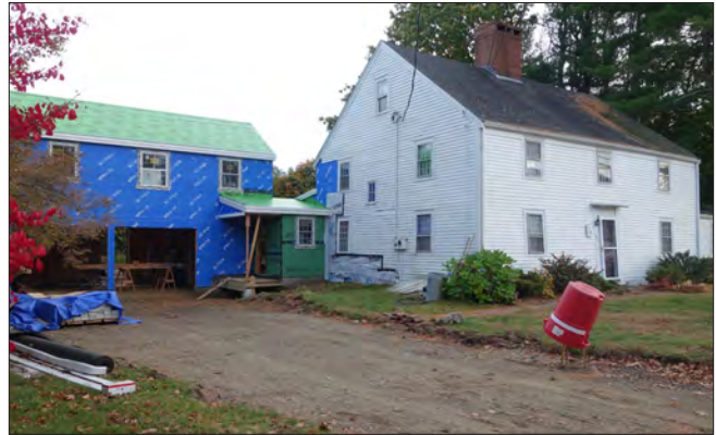
The new addition, located towards the rear, is both compatible with the historic house and contemporary in design. The smaller massing clearly identifies the addition as a secondary building. The volume, the roof slope and window openings match the historic residence.
