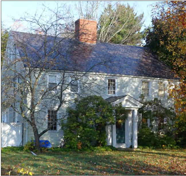
Slate roofing is often found on Rye's older buildings. Also note the massive central chimney.
